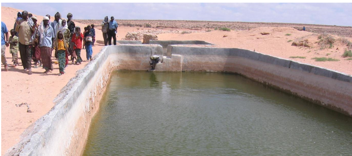
Figure 3: An example of a berkad in Somalia (Source: Banks, 2008)
