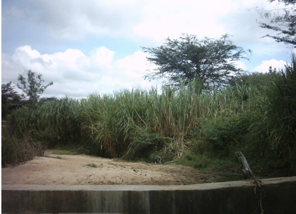
Mature sand dam Kwa Kang'esa
