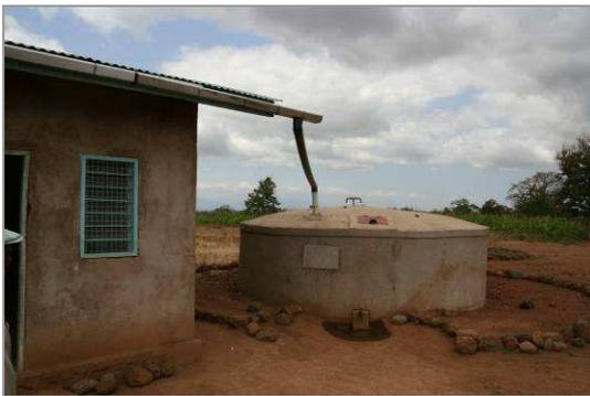
**Figure 12** Concrete tank for storage of water, collected from the roof
