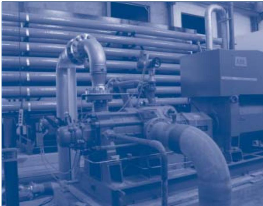
Fig. 18.11. Reverse osmosis (RO) racks and pump turbine system in La Aldea, Gran Canaria (capacity: 5000 m<sup>3</sup>/day; commissioned in 2001) (photograph by Jose M. Veza)
