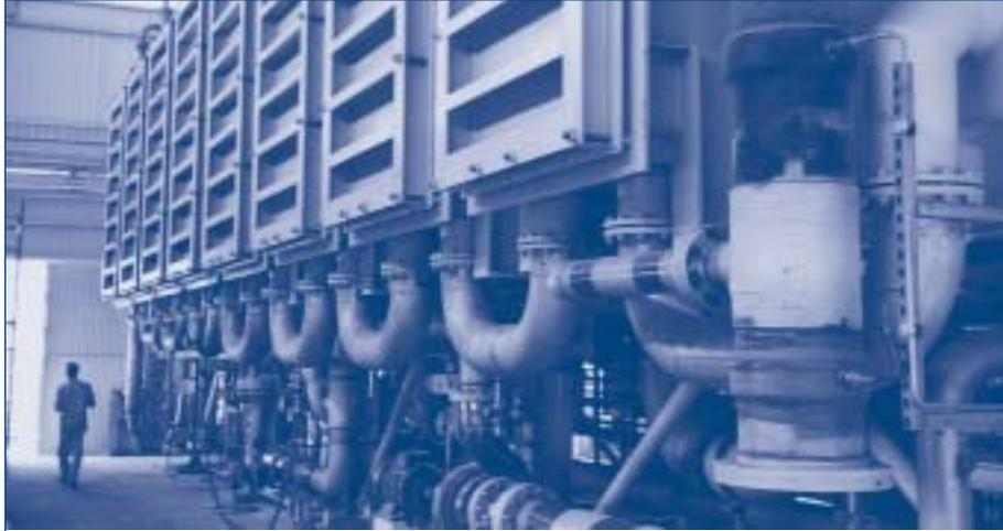
Fig. 18.2. Multi-effect distillation plant with vapour compression (MED +VC) in Mindelo, Cape Verde (capacity: 2400m<sup>3</sup>/day) (photograph by Jan C. Schippers)
