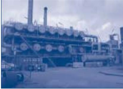
Fig. 18.4. Multi stage flash (MSF) distillation plant, Las Palmas, Gran Canaria (capacity:  $2 \times 9,000 \text{ m}^3/\text{day}$ ; commissioned in 1980) (photograph by Jose M. Veza)
