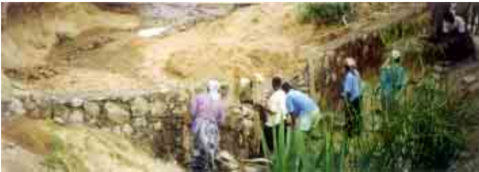
Plate 5: Building a sand dam of rubble stone masonry.
