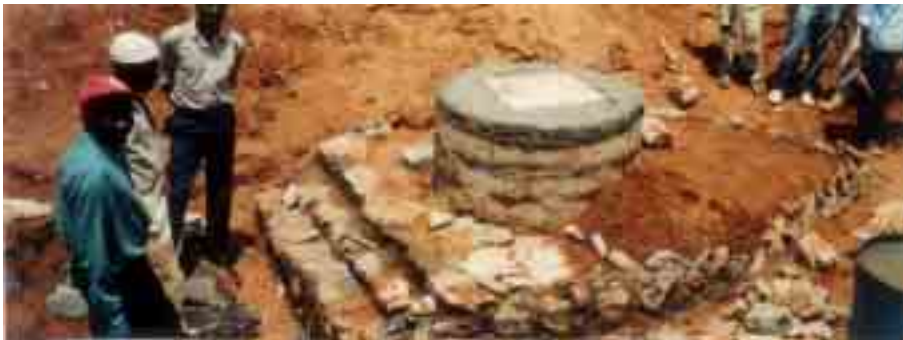
Plate 2: A hand-dug well with a hydrodynamic well head being build.
