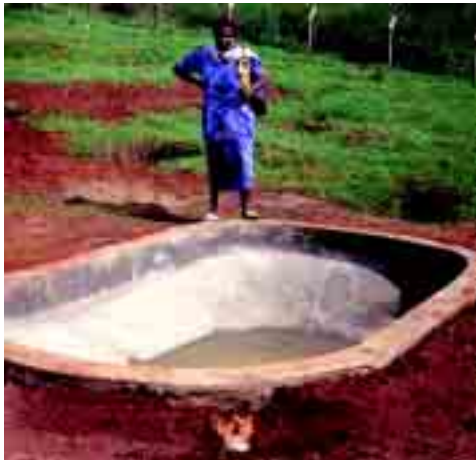
Plate 3.3 Oval tank lined with cement-sand mortar reinforced with sisal.
