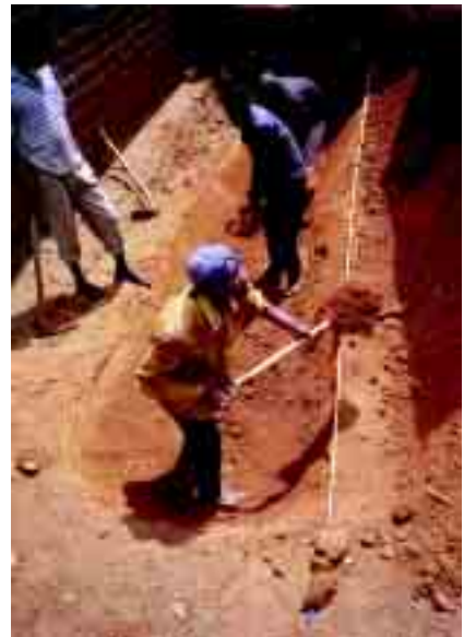
Plate 3.4 Layout and excavation of sausage-shaped tank.
