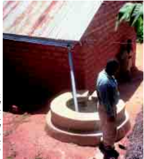
Plate 3.2 Completed ceramic tank after back-filling and construction of the neck with brickwork.
