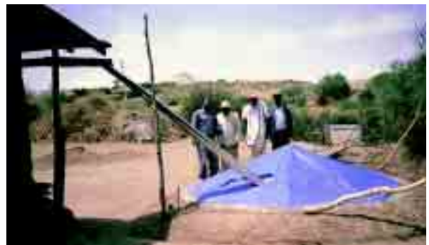
Plate 2.4 Completed tank with gutters and delivery pipe installed.
